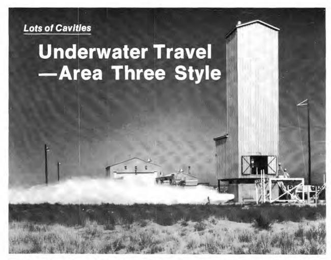
RUNNING full blast with a six-inch diameter stream of water traveling at 450 fps, the water tunnel facility sprays water across the mesa in Area III.
